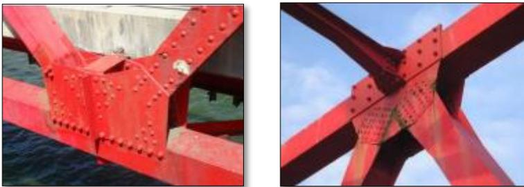
Fuente: Compressive loading test of corroded gusset plate connection in steel truss bridge, Murakoshi ([https://www.pwri.go.jp/eng/ujnr/tc/g/pdf/27/27-5-3\\_Murakoshi.pdf](https://www.pwri.go.jp/eng/ujnr/tc/g/pdf/27/27-5-3_Murakoshi.pdf)).
