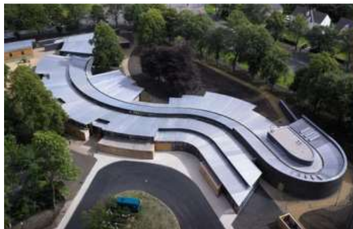
Figura N°03: Fachada Solarcity Kindergarden
