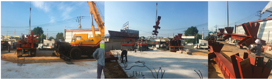
Figure 8. Transportation of the steel frame members to the laydown area.
