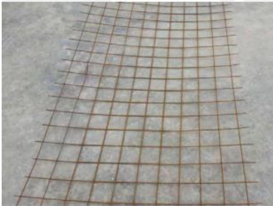
**Figura 3.18: Malla Electro-soldada - Prodac**
