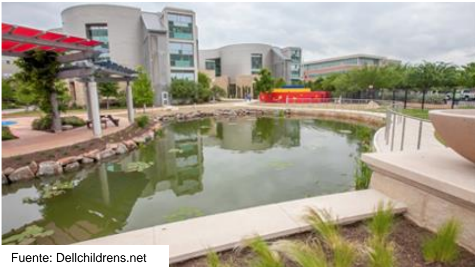
Vista frontal del hospital
