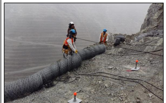
Personal realiza descenso, guiando a la malla Steel Grid.
