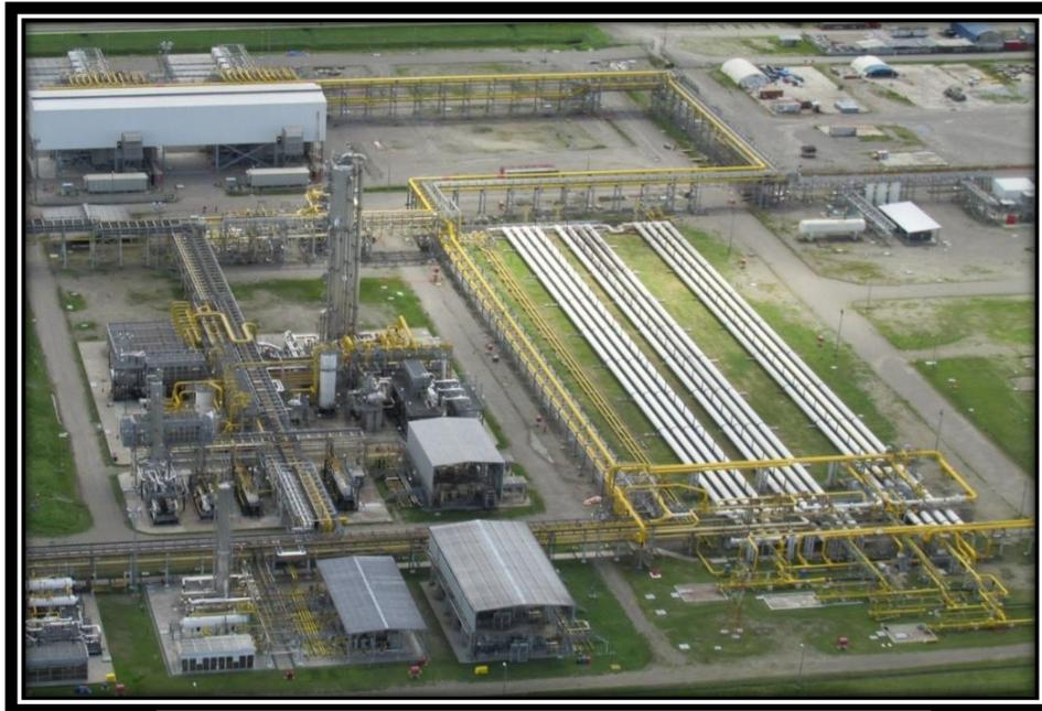
*Figura 13: Slug Catcher – Planta de gas Malvinas*
