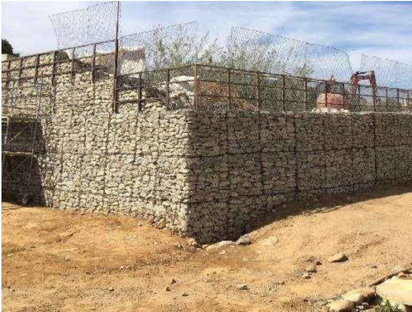
Figura 00. Terramesh System, TDM S.A .Perú 2018, Tomado de https://www.maccaferri.com/terramesh-for-retaining-walls-and-bridge-abutments-corsica/
