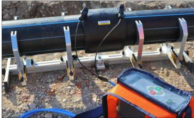
Figura 27: Electrofusion.
